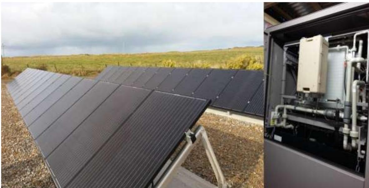
Figure 1. The 11 kW Solar PV and 40 kWh Vanadium battery system at the Each Leim site.<sup>1</sup>
